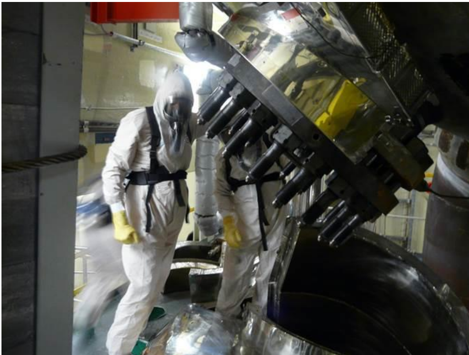
Figure 6-14 Inspection of a steam generator at the nuclear facility in Borselle, the Netherlands.
